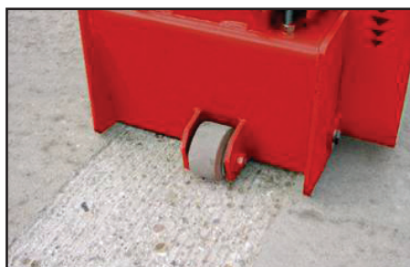
ROUGHENING CONCRETE
