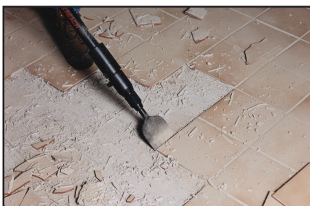
CERAMIC TILE REMOVAL
