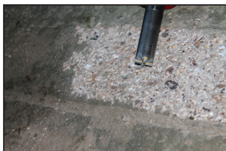
ROUGHENING CONCRETE
