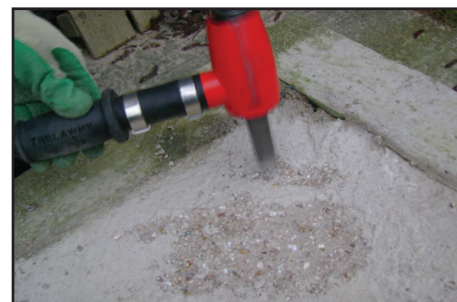
CONCRETE PREPARATION
