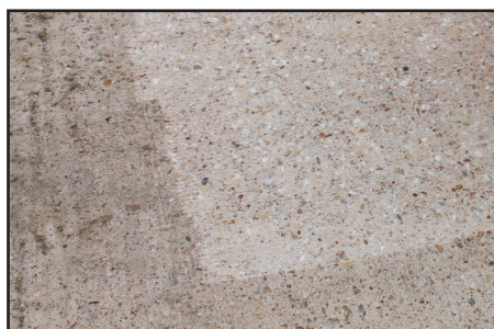
ROUGHENING CONCRETE
