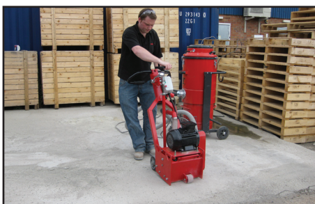
REDUCING LEVELS ON CONCRETE
