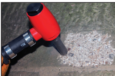
REDUCING LEVELS ON CONCRETE
