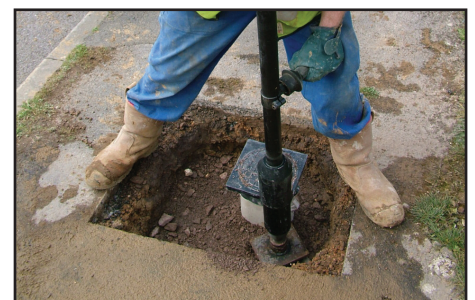
REINSTATEMENT COMPACTION
