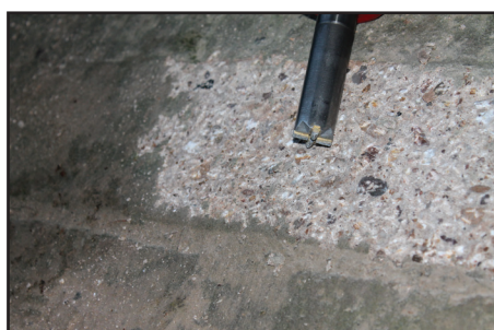
ROUGHENING CONCRETE
