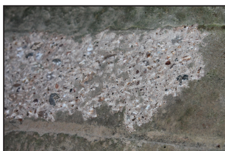
ROUGHENING CONCRETE
